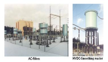
fig. HVDC Smoothing Reactor
