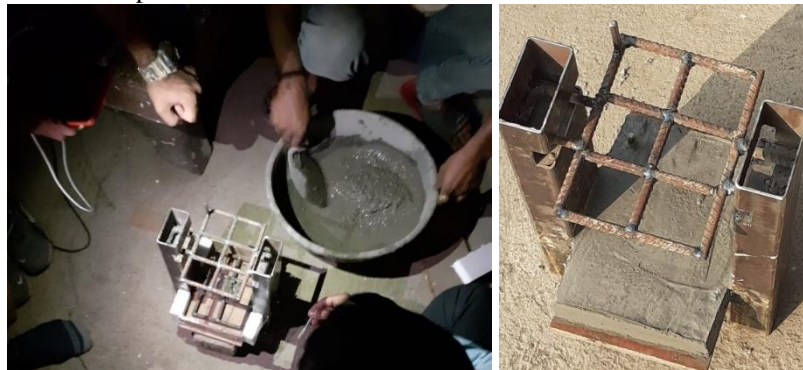
(Figure 2.2 Concrete Structure on TMT Bars and MS Pipe)
