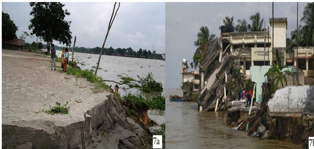
Fig. 7. People Lost Their Home and Personal Properties During Flood After Breaking River Embankment 2017 (Newspaper Daily Sun 28/07/2017).
