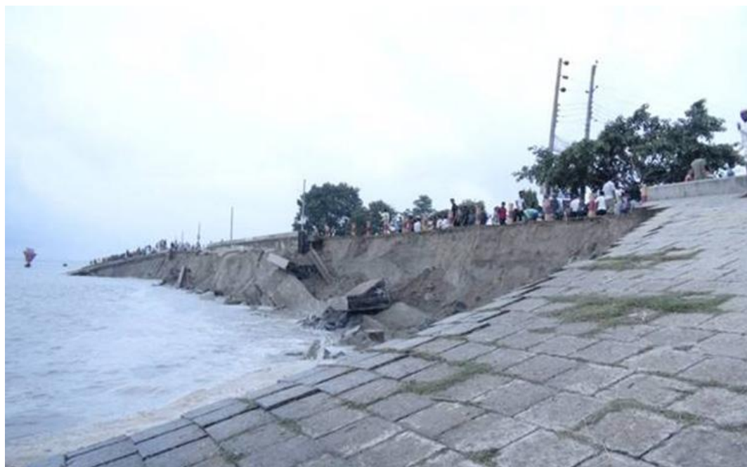
Fig. 3. Food Breaks River Embankment Which Is Made by Only Concrete Block and Soil.
