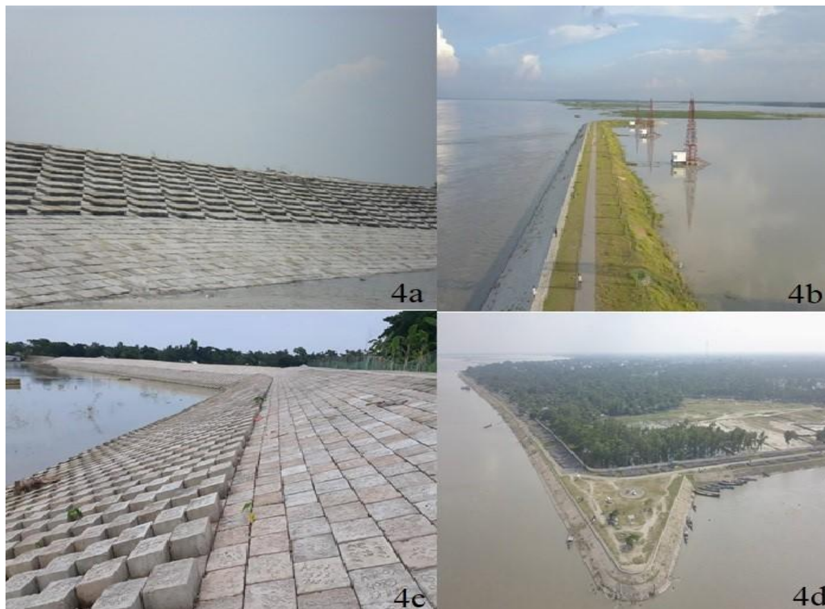
Fig. 4. Newly developed Jamuna and Padma river embankment maintaining proper slope stability factor of safety.
