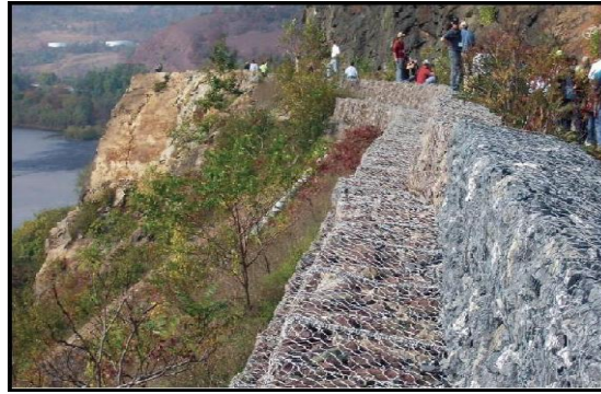
Fig. No.9: Gabion wall
