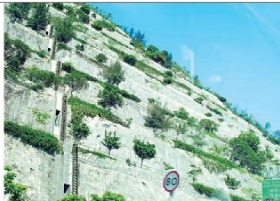
Fig. No. 12: Slope stabilization using vegetation
