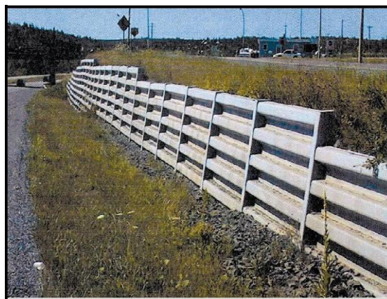
Photograph No.8: Steel bin wall
