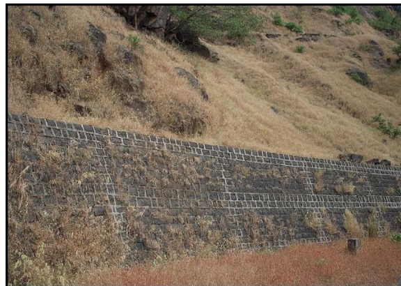
Fig. No.6: Rock-fill buttresses
