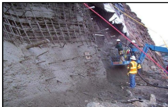
Fig. No. 14: Shotcrete operation.
