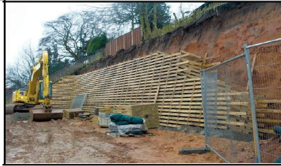
Fig. No. 7: Timber crib wall
