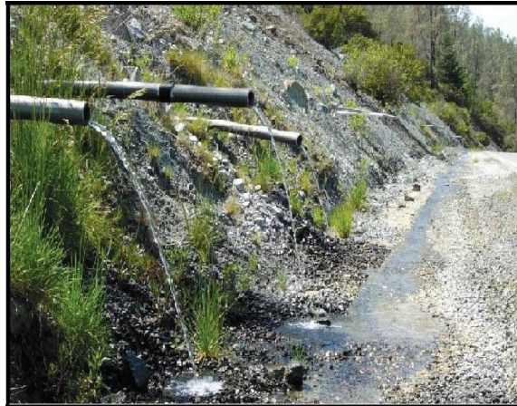
Fig. No. 11: Subsurface drainage.
