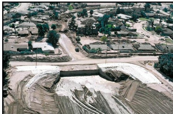
Fig. No. 16: Debris-flow basin
