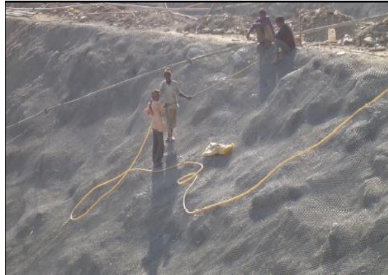
Fig. No. 5: Plastic mesh reinforcement
