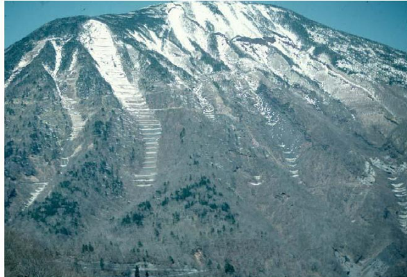
Fig. No. 13: Check dams
