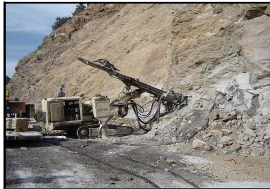
Fig. No. 15: Rock bolting operation
