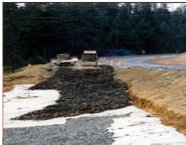
Fig. No. 4: Backfilling lightweight material
