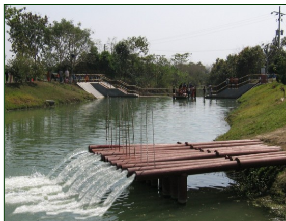
Figure 5: Use of Surface and Rain Water for Irrigation
