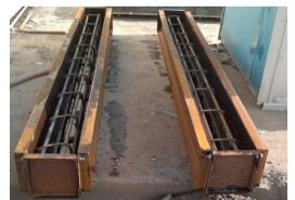
Photo (1) Steel moulds for casting the all reinforced concrete beams.
