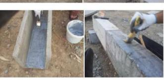
Photo (4) Methods of casting and fixing the ferrocement sections.
