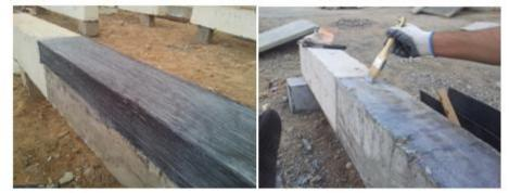
Photo (5) Method of rehabilitate the damaged beam using carbon fiber.
