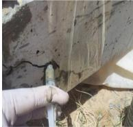
Photo (7) Beam during repairing using the injection technique.
