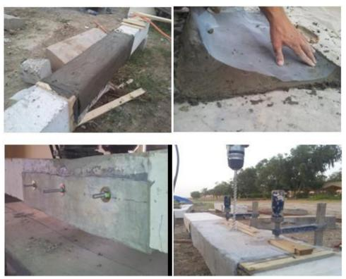
Photo (6) Casting and fixing the developed nano ferrocement section.
