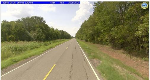
Figure 3: Pavement distresses [Source DOTD]
