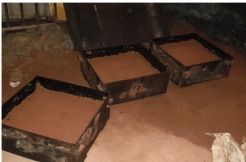
Figure 3: Casting stage of compressed stabilized laterite slab
