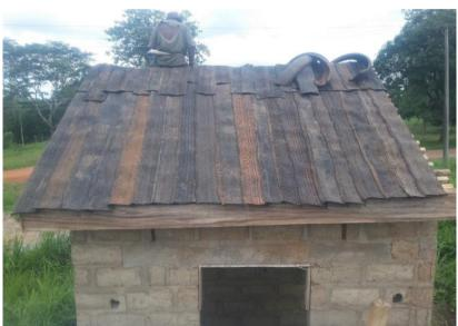
Plate1: The Constructed Tyre Roof
