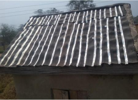
Plate 2: Tyre Roof with Flash Band Adhesive to Prevent Leakages
