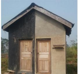
Plate 3: The house roofed with used tyres
