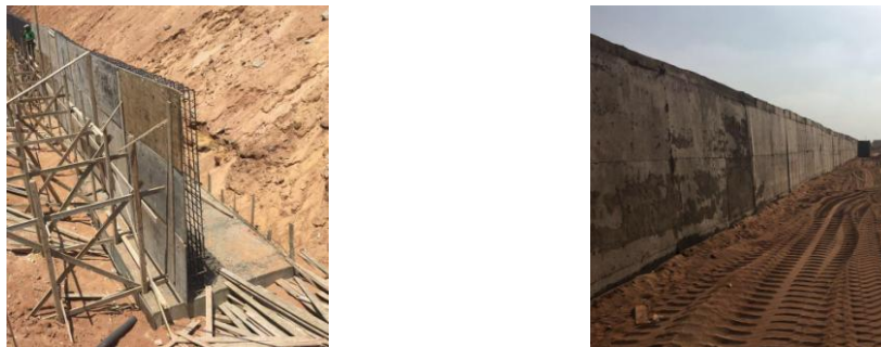
Figure 4: Fixed reinforced concrete fence.
