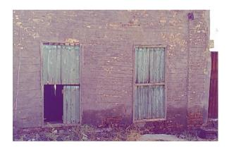
Photo(10)Shows old traditional windows style in Almaden quarter buildings ,and it has rectangular shape with wooden frame. Source :add by author
