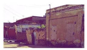
Photo(8)Shows walls falling down in Almadneen quarter buildings ,because absence of using modern technology in it. Source :add by author
